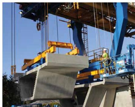
*The launching truss moves guideway segments into position on the northeast corner of Como Lake Avenue and Clarke Road in Coquitlam.*
