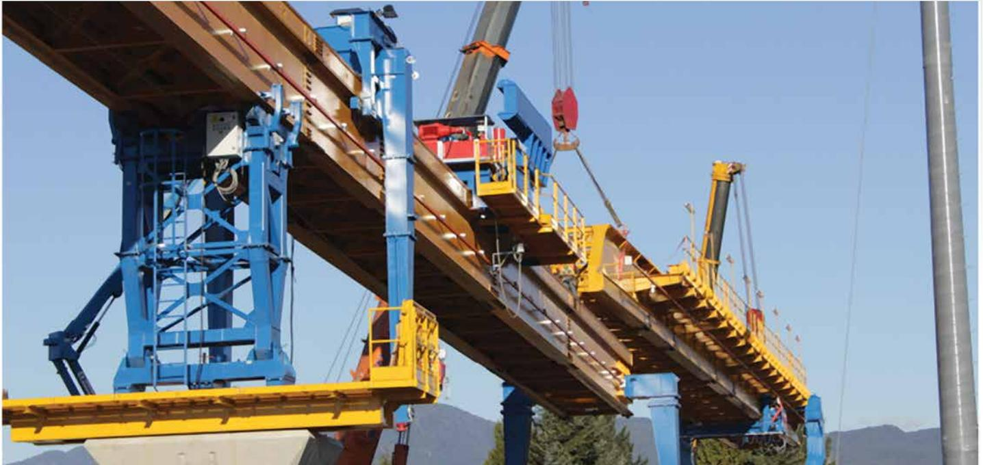
*The launching truss is assembled in Burquitlam to prepare for the installation of the first elevated guideway segment.*
