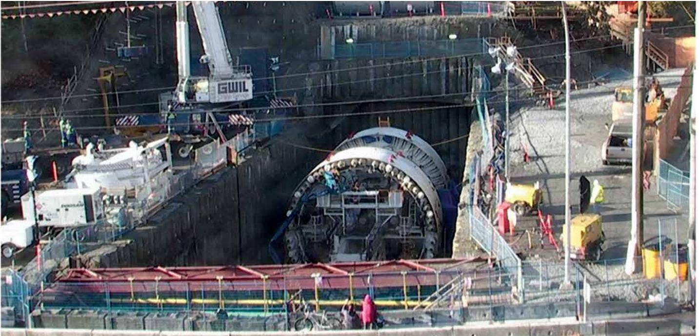
Assembly of the tunnel boring machine is taking place at the north tunnel portal launch site.
