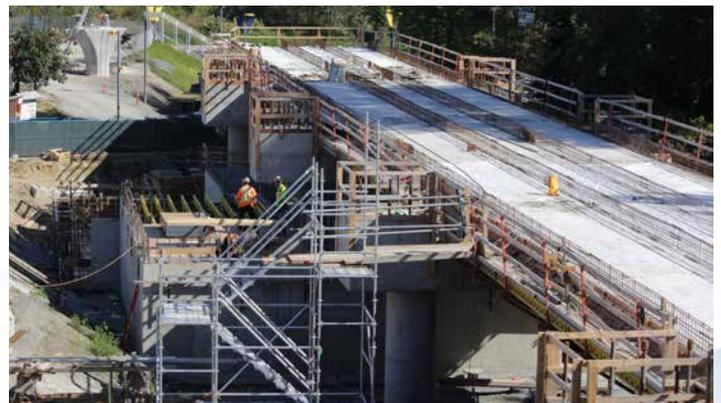
Coquitlam Central Station construction has seen installation of girders and internal structures. The Evergreen Line launching truss will be assembled in this area to start elevated guideway construction along Pinetree Way.
