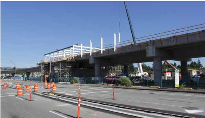
The elevated guideway has been completed through Burquitlam Station. The steel frame of the station is above the guideway.
