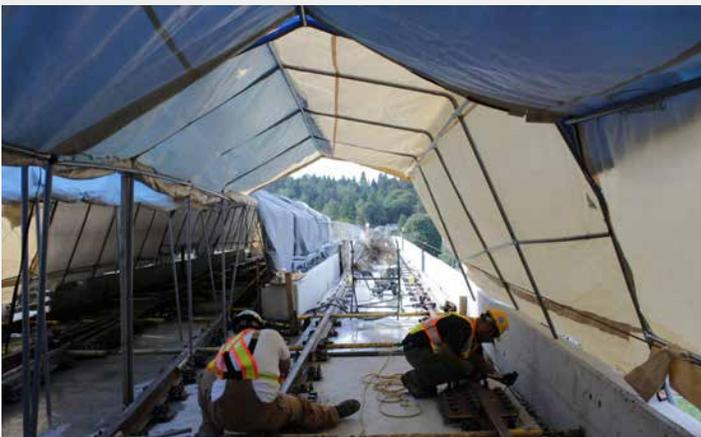
*The track work crew installing rails on the elevated structure by Schoolhouse Creek in Port Moody.*
