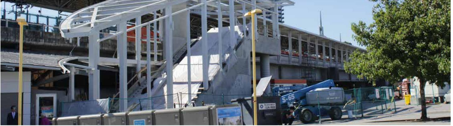
The new entrance for the Evergreen Line at Lougheed Town Centre Station is taking shape. The structural steel has been installed to support the glass roof over the stairs and escalator.
