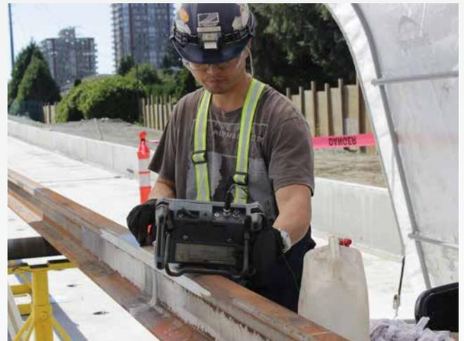
At a rail welding operation at the south tunnel portal in Burquitlam, quality control includes the use of ultrasound technology to inspect each weld.
