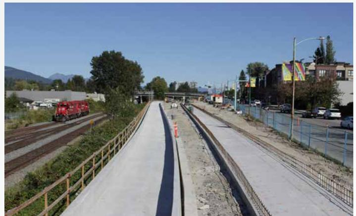
*The Evergreen Line at-grade guideway between the existing rail line and Clarke Street in Port Moody. The guideway passes under the Moody Street overpass on the way to Moody Centre Station.*
