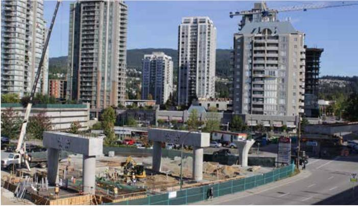
Foundation work is underway at Lincoln Station, and the support structures are ready for the launching truss to come through to install the elevated guideway.
