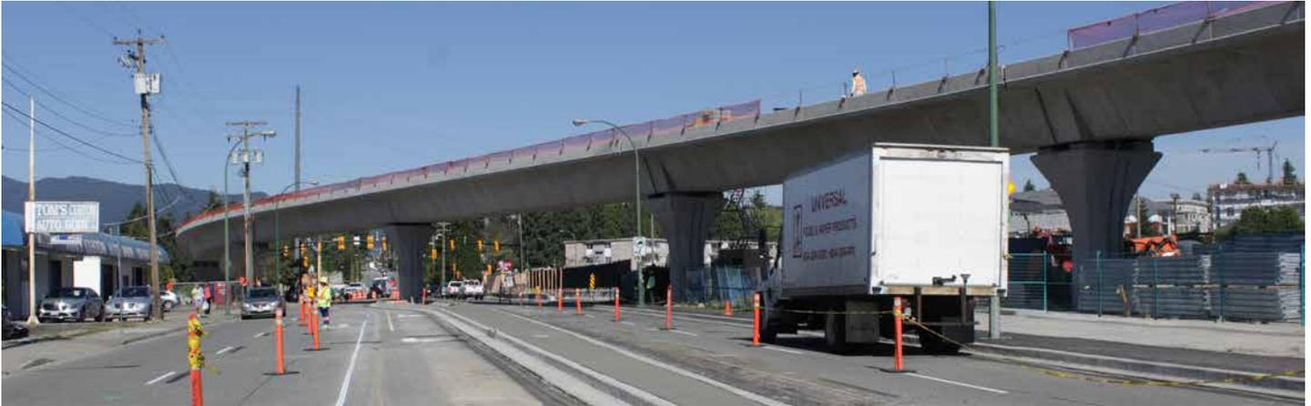
*With the completion of the elevated guideway structure, roadwork crews have moved in to do final road work. On Clarke Road in Burquitlam that includes new medians, sidewalks, signal work and repaving.*
