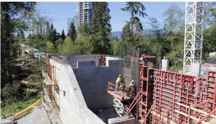
At Inlet Centre Station construction crews are busy installing reinforcing steel at the west entrance to prepare for a concrete pour for the station way. To watch the construction, check out the webcam on the project website.
