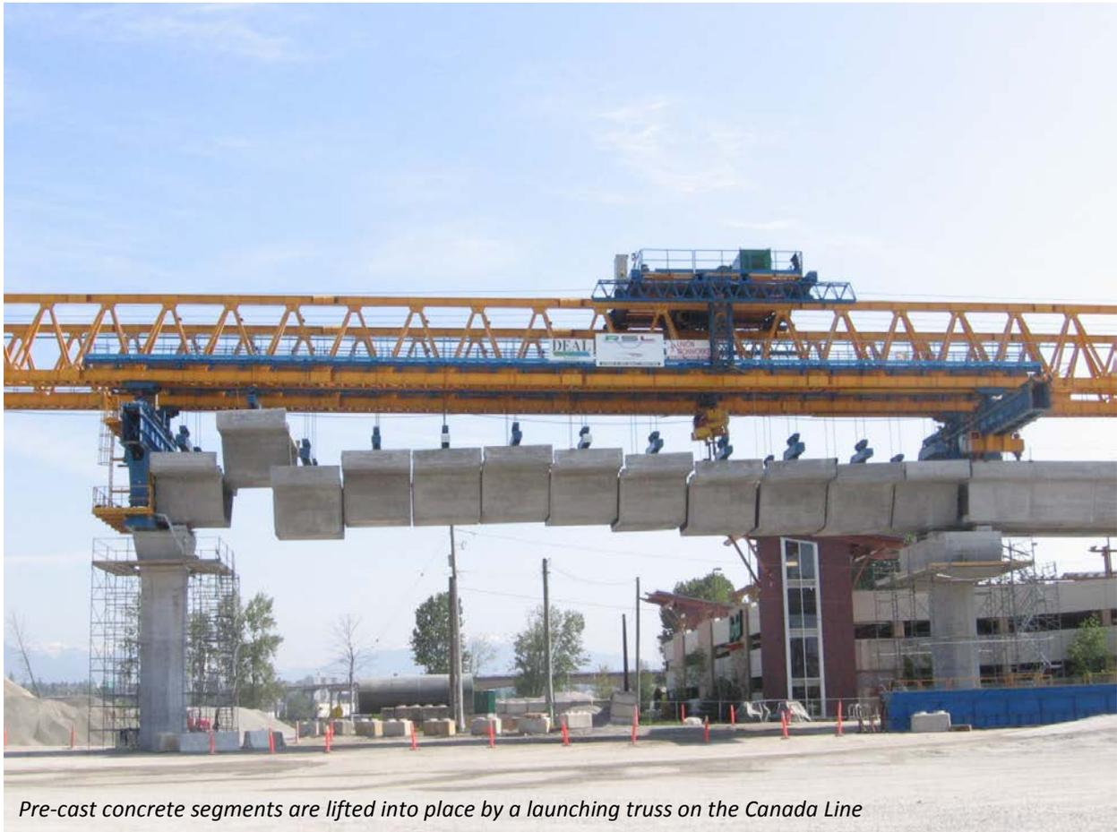
*Pre-cast concrete segments are lifted into place by a launching truss on the Canada Line*
