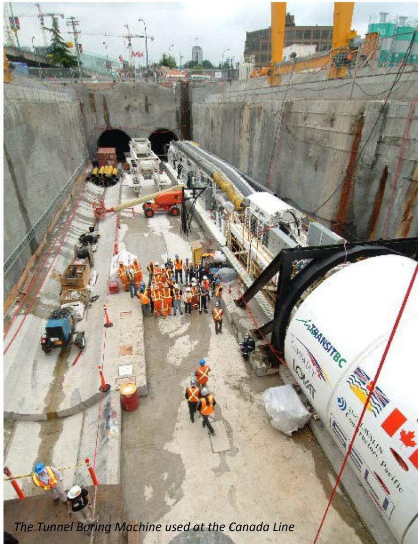
*The Tunnel Boring Machine used at the Canada Line*
