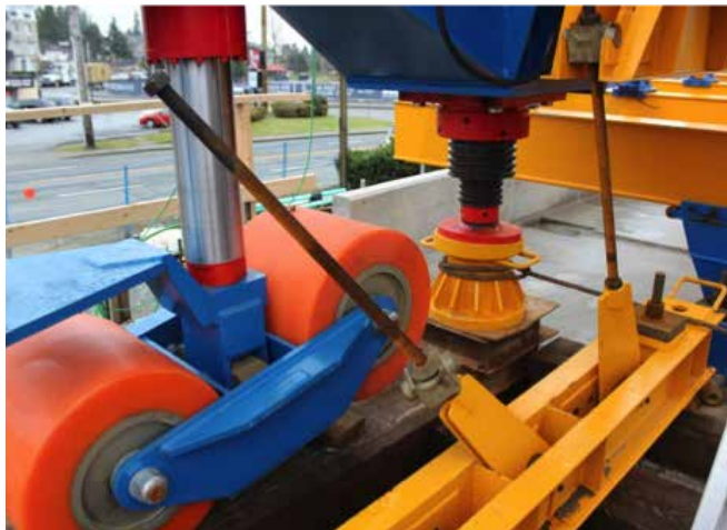
Left: Once a span is complete, the launching truss can be rolled ahead on the new guideway. Right: The launch truss forward leg is moved to the next column top.
