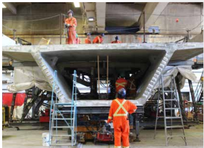
Guideway segments are manufactured in Richmond by Armttec.
