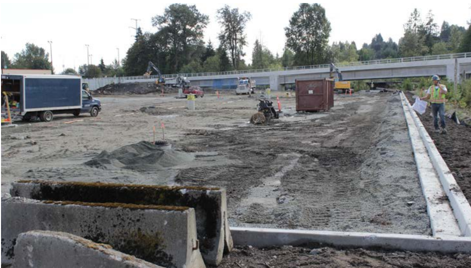
Park and Ride construction at Coquitlam Central Station
